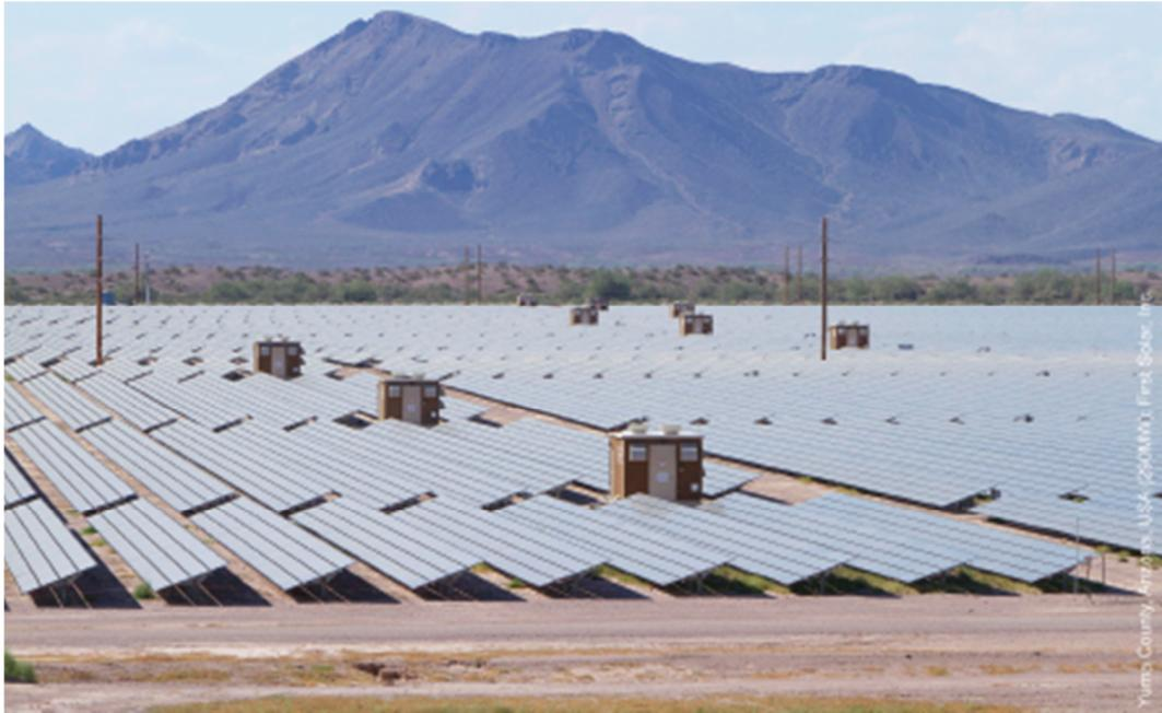
Figure 34: First Solar's Yuma County-Arizona, 290 MWp CdTe PV power plant with grid-friendly plant control [67].
