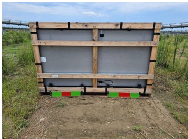
Figure 2: Correct Engagement Points for Lifting Pack from Long Side
