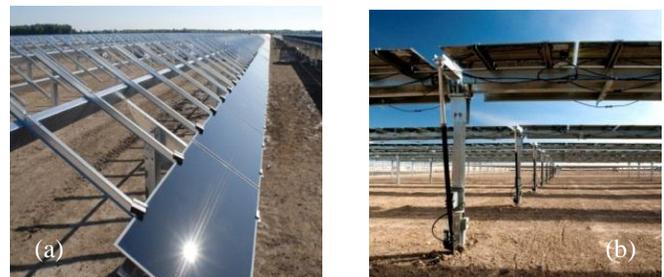
Fig. 2: Mounting structures for (a) fixed-tilt and (b) single-axis horizontal tracking utility-scale CdTe PV systems.
