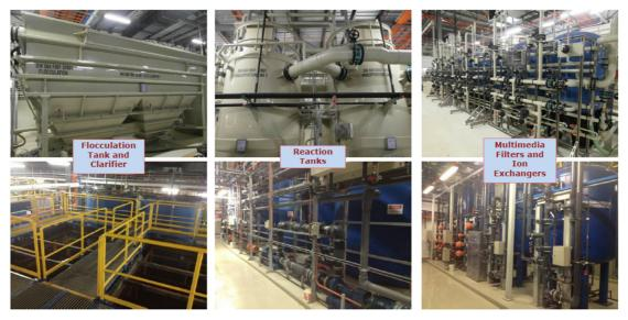
Figure 28: Equipment used at First Solar's dedicated wastewater treatment plant.
