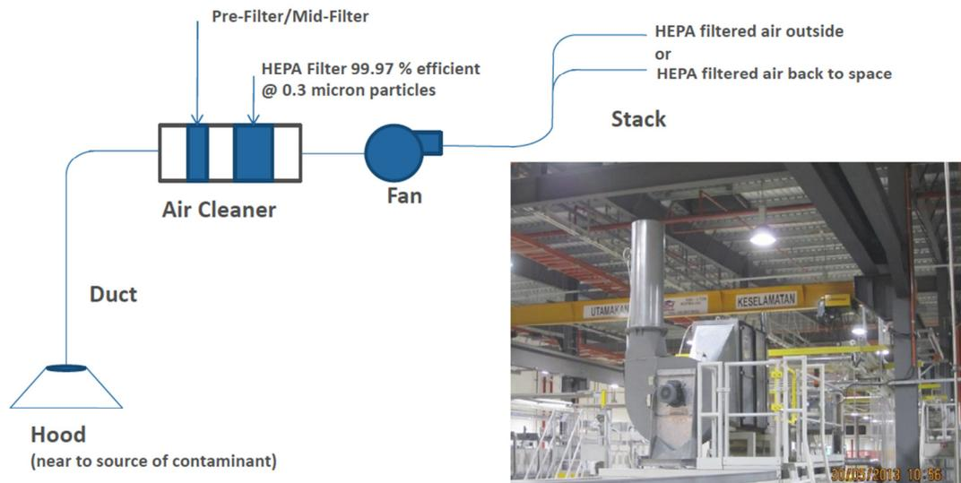
Figure 24: First Solar's CdTe PV module manufacturing plant Local Exhaust Ventilation (LEV) system. The photo shows the High Efficiency Particulate Air (HEPA) filter's exhaust air being recirculated back to the manufacturing floor space.
