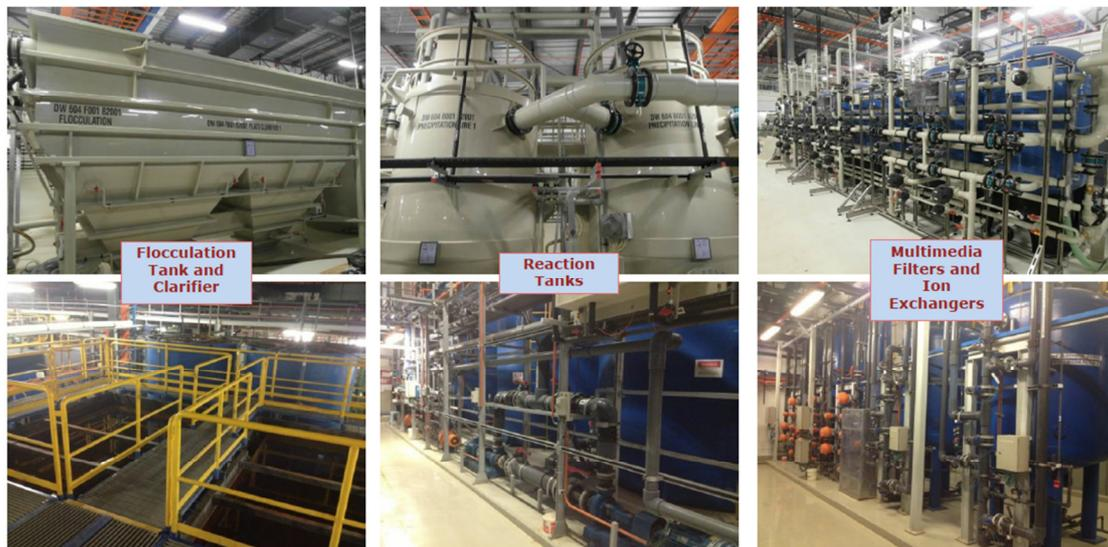
Figure 28: Equipment used at First Solar's dedicated wastewater treatment plant.
